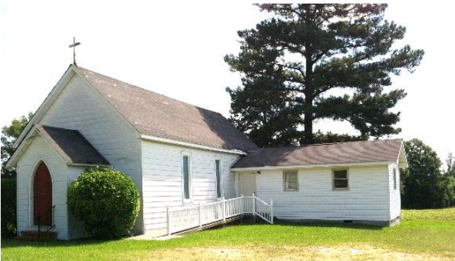
St. Anna's Episcopal Church, Littleton (1894 - 2007) SR 1404 (Bacon Road), Littleton, Diocese of North Carolina Photo: 1904 building and addition
