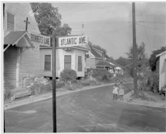
St. Andrew's Episcopal Church (1909 – 1970) Formerly on Bonners Lane in Greenville, Diocese of East Carolina Photo: courtesy Joyner Library, East Carolina University
