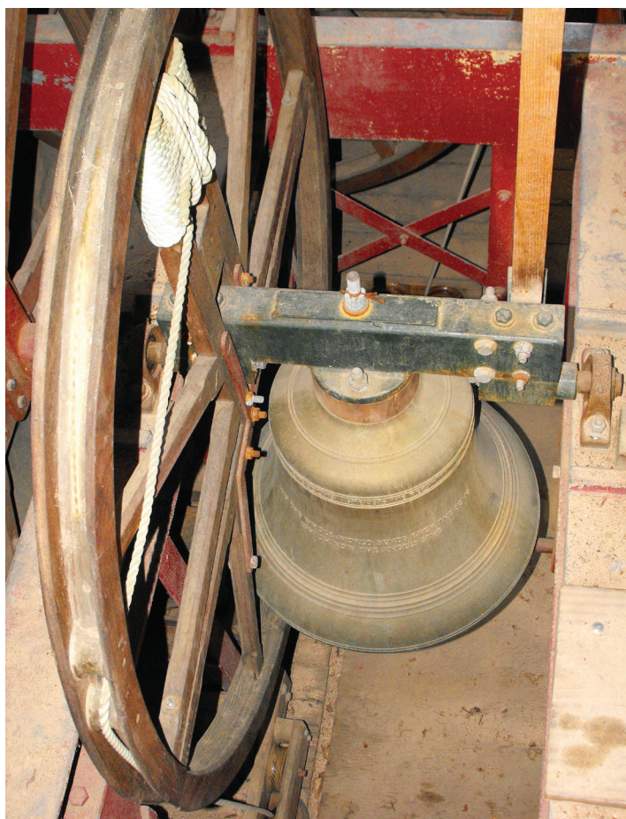
Change ringing bells hang freely from a pivot point. The rope, which runs down through the ceiling, turns the wheel, which rotates the bell in a complete circle and allows the clapper to catch both edges of the bell’s opening, which means the bell rings regardless of the direction in which it is rotating.
